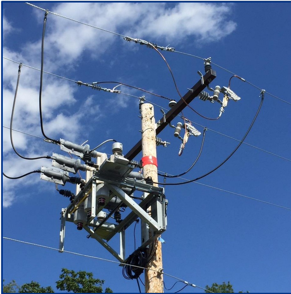
Protective & Sectionalizing: Vacuum Circuit Recloser
