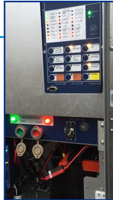
Recloser Control with Downed Conductor Detection
