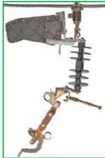
Sectionalizing: Load-Break Switch
